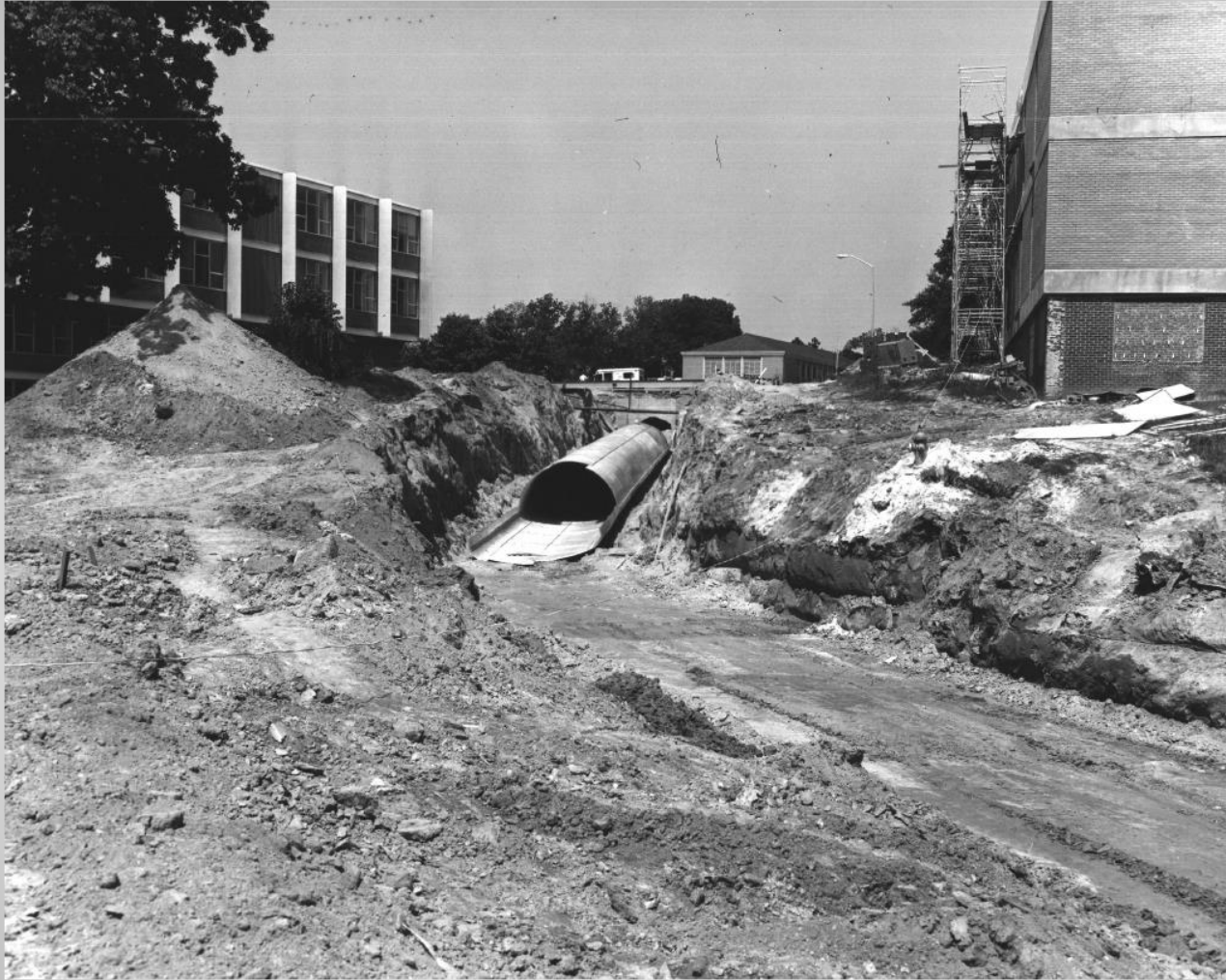
1965 STEAM & ELECTRIC DISTRIBUTION TUNNEL CONSTRUCTION
