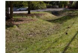
Closer view of the swale and how it directs water
