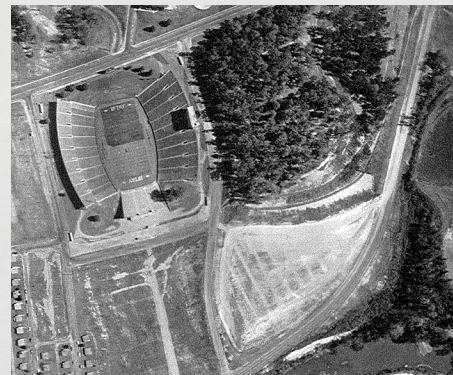
Right: 1963 Aerial Photograph, courtesy Campus Facilities. The parking lots South of the cemetery have been graded.
